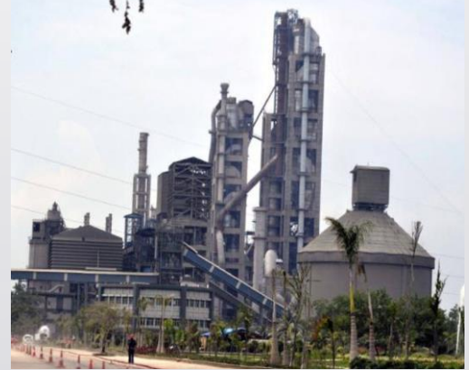
Figure 3: Cement Manufacturing Company [3]
